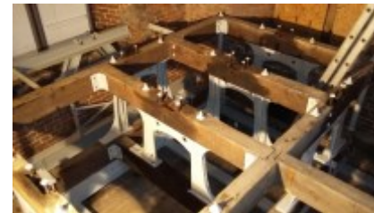
The restored bell frame, ready and waiting!
